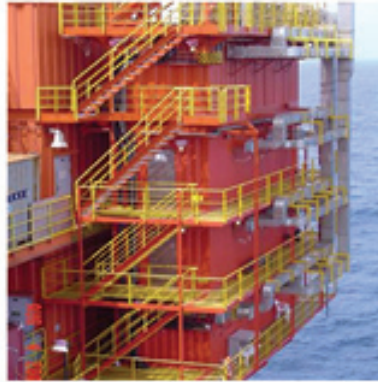
Project : Additional Offshore Living Quarters, Yadang Platform Client : Premier Oil Myanmar Ltd.
