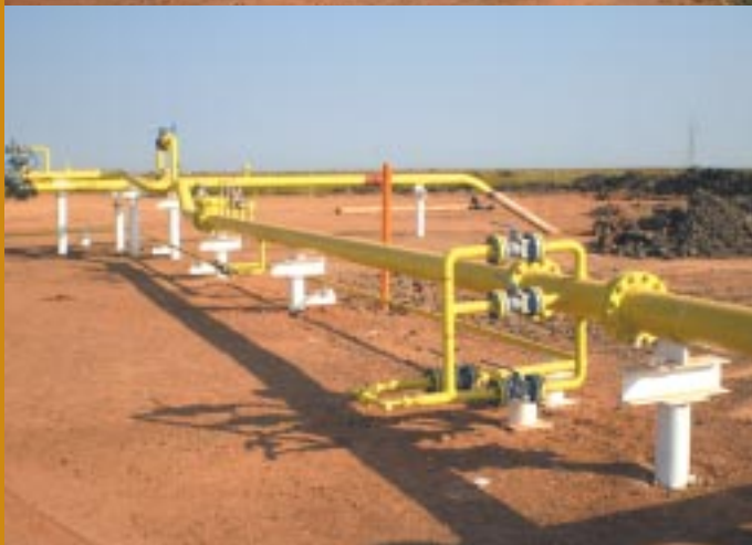
Mala Satellite – Wellhead - above ground piping
